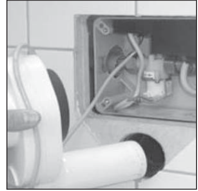
Insert sensorsiphon
